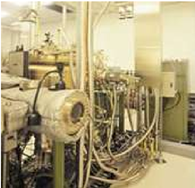
Piping to a typical MBE hook-up
