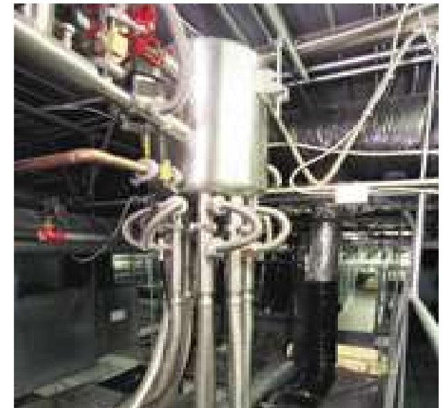
Liquid Vapor Phase Separator
